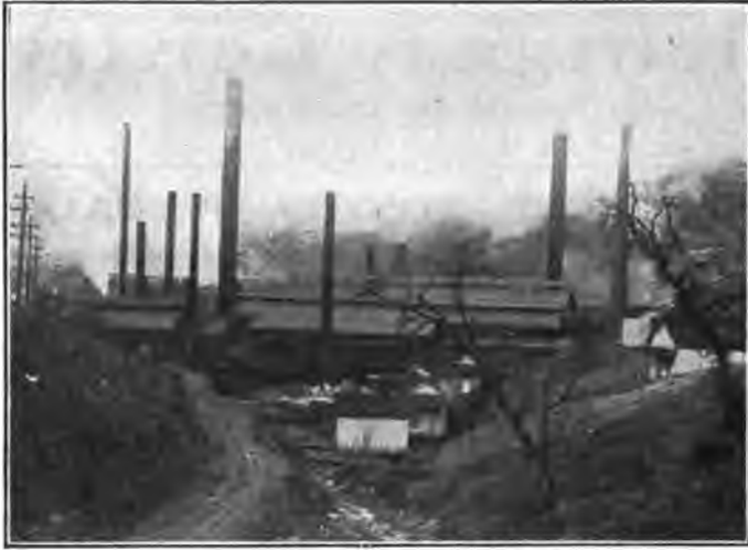
Mountain Copper Co. Smelter, Keswick, Shasta Co., California.
